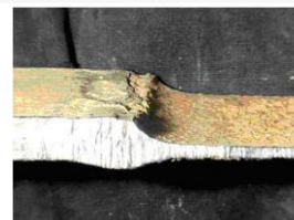
Figure 5-5 – Cross-section of a carbon steel pipe showing preferential corrosion of the pipe with high residual element content on the right (%Cu + %Ni + %Cr), as compared to the low residual pipe section to the left of the weld.
